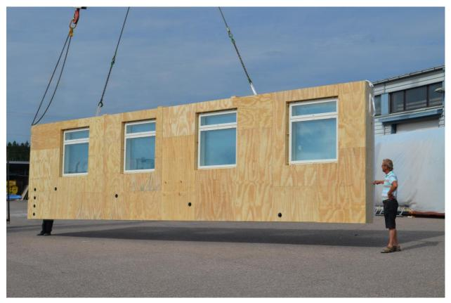
Fig. 3 The elements are transported in horizontal position and will be turned by the crane. The model element was tested at the element factory before the manufacturing was started. The round holes are the ventilation ductwork connections. Photo: Kimmo Lylykangas.
